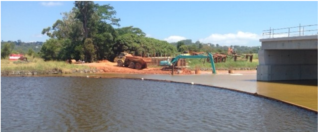
Class 2 Premium Silt Curtain installed in tidal river.
