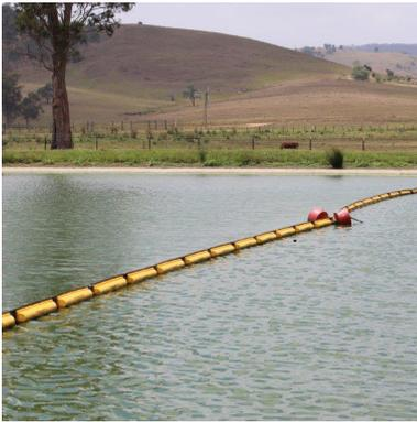
The purpose of a Floating Baffle is to improve the operating efficiency of a waste water treatment system. These systems may make up part of a sewage treatment plant, industrial waste water treatment plant or other treatment processes related to mining or the oil and gas sectors.
