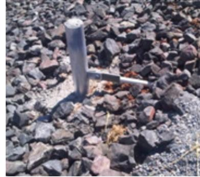
A Dead Man Anchor or an Anchor Post secured by concrete and dug into the embankment are the most common approaches. These bank moorings can be further reinforced using either a Screw Anchor or a Flat Plate.
